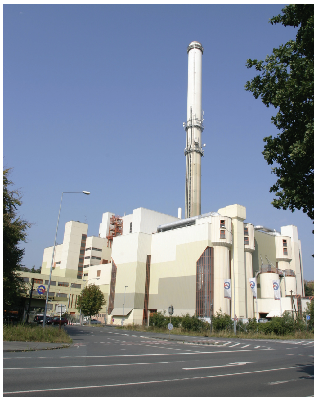
MVV's CHP plant in Offenbach, Germany which processes 250,000 tonnes of waste
